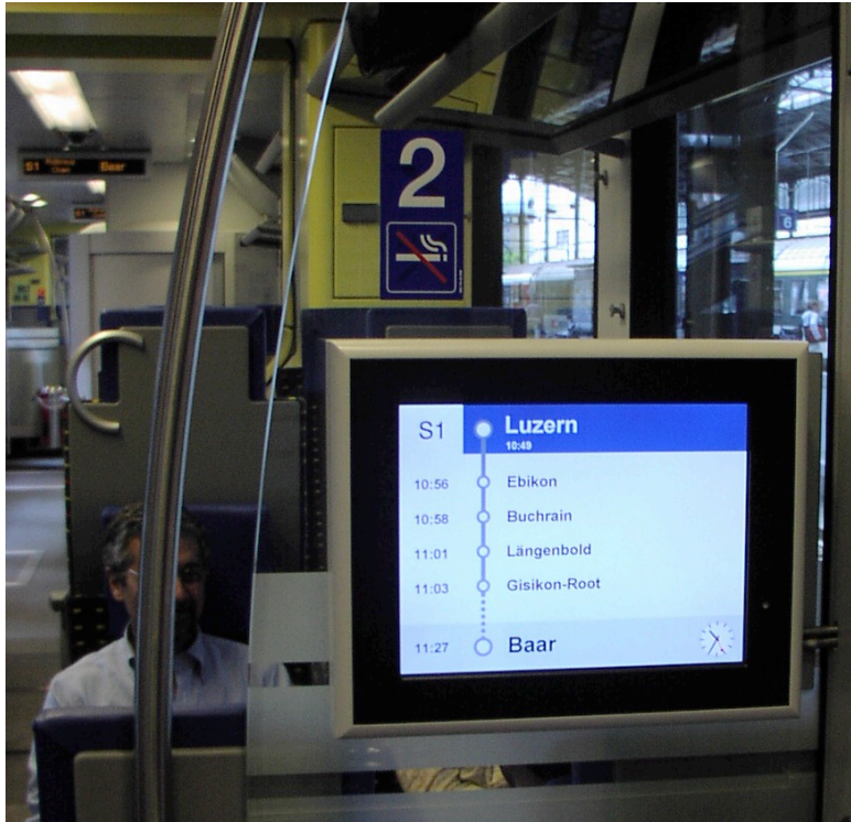
FIGURE 5 – Stadtbahn Zug passenger information video display.
